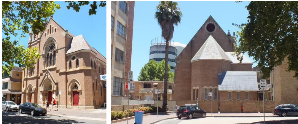
Figure 60 – Leigh Memorial Uniting Church, showing the North Elevation facing onto Macquarie Street (left) and South Elevation backing onto Civic Place (right) (Source: NBRS+PARTNERS, January 2013)
