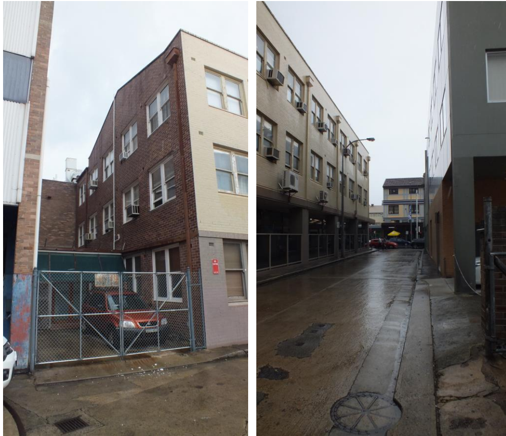
Figure 53 — Left: view from United Lane showing the north elevation of the building located on the subject site at No 48 Macquarie Street. Right: view south along United Lane to the intersection with Macquarie Street, with the subject site shown to the left. (Source: NBRSPARTNERS, April 2015)
