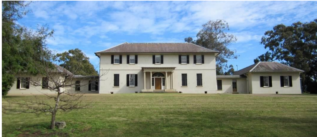
Figure 63 – Old Government House, East Elevation, showing the Main Entry portico (Source: NBRSPARTNERS, Sept 2012)
