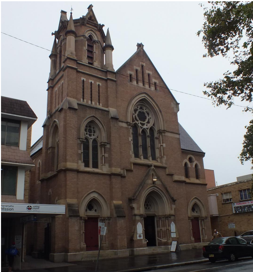
Figure 50 — Leigh Memorial Uniting Church, located at 119 Macquarie Street, is a heritage item on the southern side of the street and southeast of the subject site (Source: NBRSPARTNERS, April 2015)
