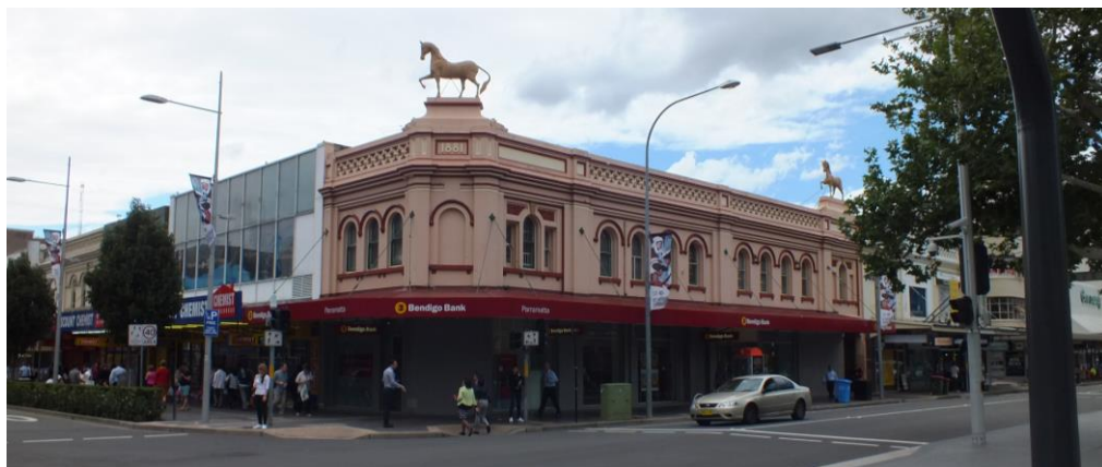
Figure 33 — View to the eastern-side of Church Street, at the corner of Macquarie Street. Buildings along both streets are predominantly three-storey in height (Source: NBRS+PARTNERS, April 2015)
