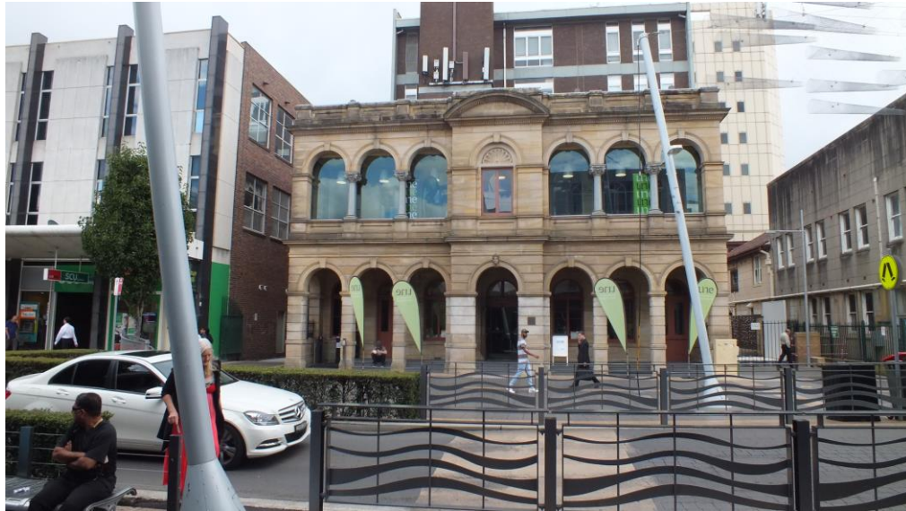
Figure 38 — the former post office, located at 213 Church Street, on the western side of the street and opposite the subject site, is a free-standing sandstone building dating to the Victorian period. Mid-twentieth century buildings adjoin the building to the south and west (Source: NBRS+PARTNERS, April 2015)
