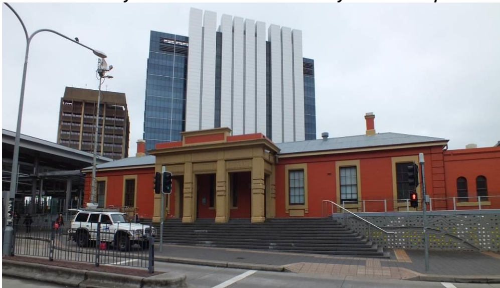
Figure 58 – Parramatta Railway Station, Main Entry, located on Argyle Street looking northeast showing Parramatta CBD multi-storey office buildings in the distance (Source: NBRSPARTNERS, July 2012)
