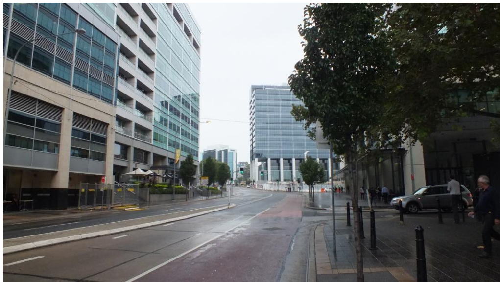
Figure 43 — View south along Smith Street showing the extent of late-twentieth century and early twenty-first century high rise development within close proximity to the subject site (Source: NBRSPARTNERS, April 2015)
