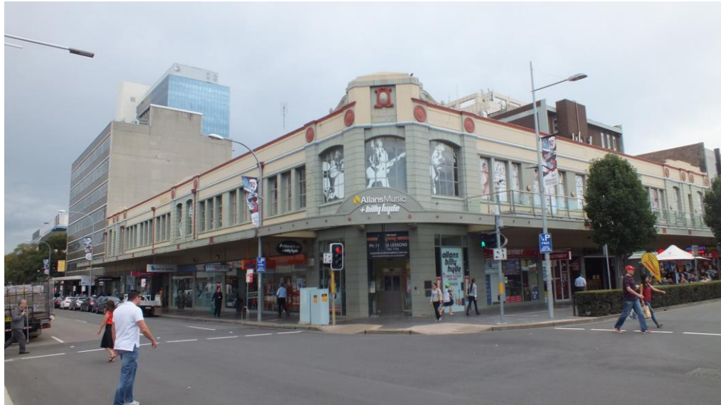
Figure 34 — View to the western-side of Church Street, at the corner of Macquarie Street showing the two-storey Murray Bros Building. Mid-twentieth century buildings are located to the west of the Murray Building and are seven storeys and above (Source: NBRSPARTNERS, April 2015)
