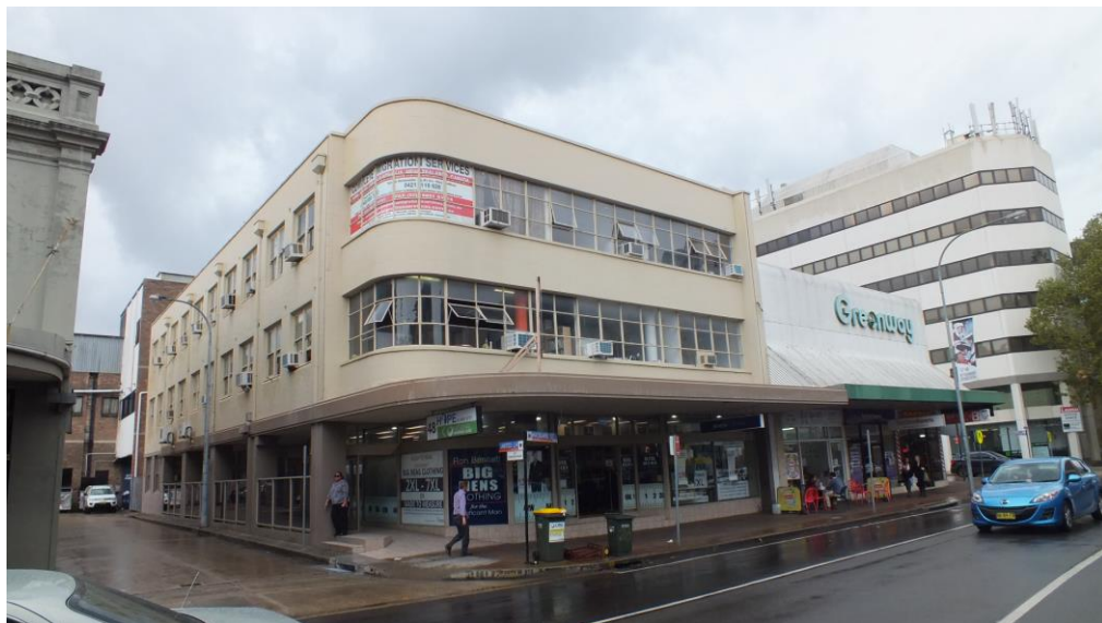
Figure 52 — View of the subject site looking north to the intersection of Macquarie Street and United Lane. The former United Insurance Building located at No 48 Macquarie Street (left) dates to the mid-1950s. The Greenway building, on the corner of Horwood Lane (right) dates to the 1960s (Source: NBRSPARTNERS, April 2015)
