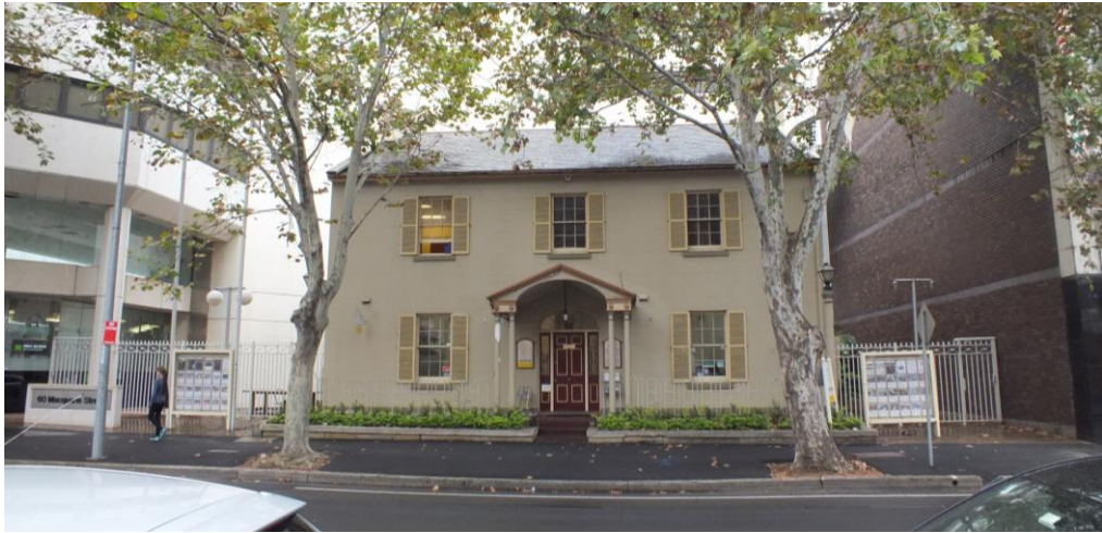
Figure 49 — Two-storey villa of Kia Ora, located at No 109 Macquarie Street, east of the subject site is a heritage item and potential archaeological site (Source: NBRSPARTNERS, April 2015)
